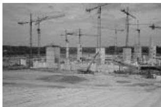
Fig. 1 A bird's eye view of the construction site
